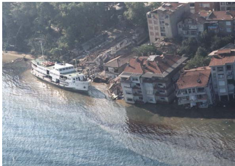
Figure 1.9: Sliding and flooding along the Gölcük coast (Kocaeli Earthquake 1999)
