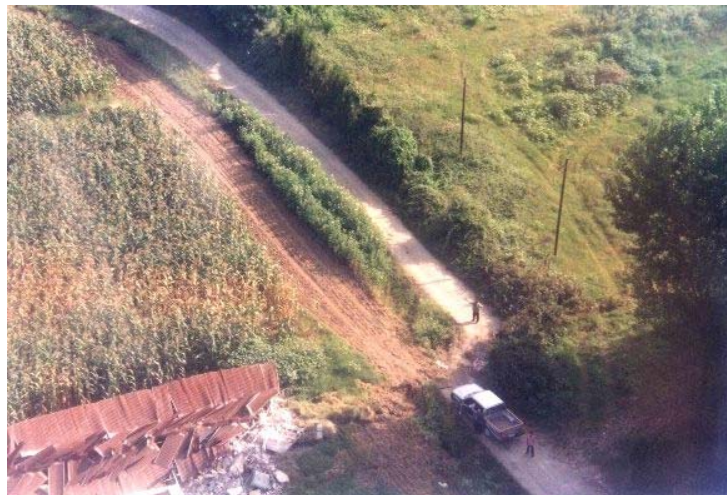
Figure 1.10: Fault rupture with lateral displacements of around 4m (Kocaeli Earthquake 1999)
