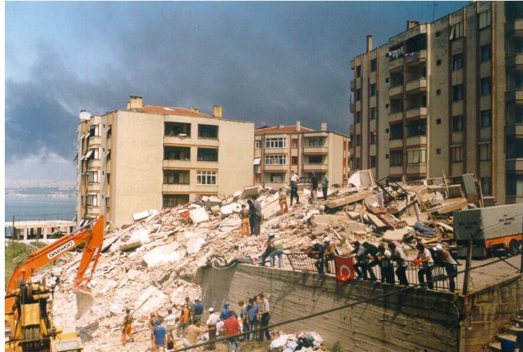
Figure 1.5: Variation of damage in Gölcük (Kocaeli Earthquake 1999). Totally collapsed building and buildings with moderate damage possibly as result of different construction layouts or site factors
