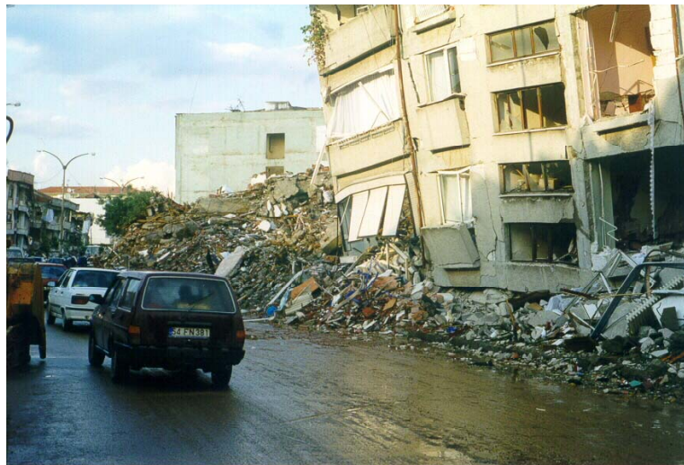
Figure 1.6: Damage in Adapazari (Kocaeli Earthquake 1999). Collapse of soft story
