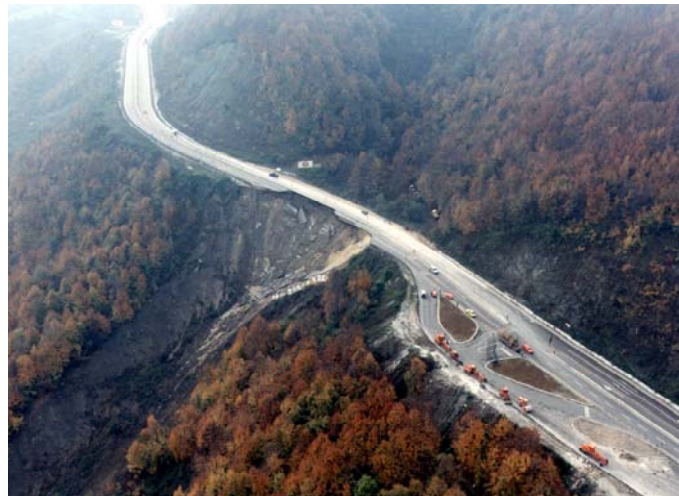
Figure 1.8: Slope failure along the Istanbul-Bolu highway (Duzce Earthquake 1999)
